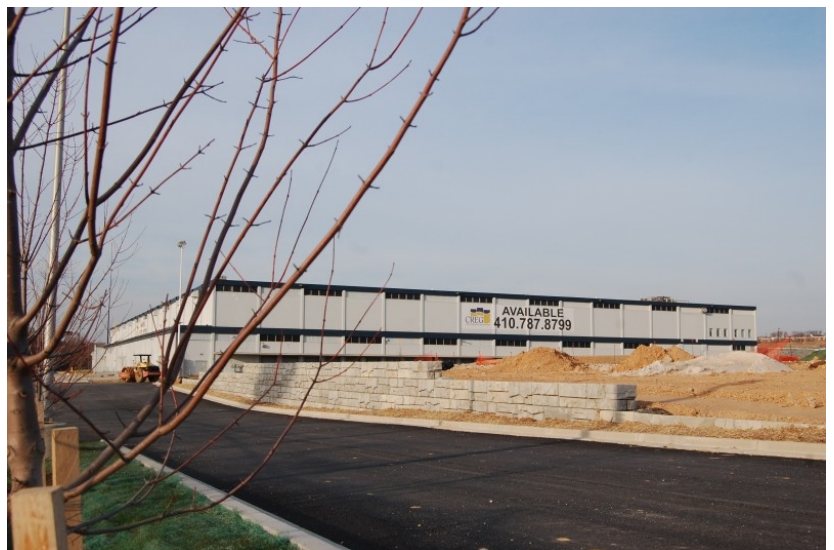
Port 95 Industrial Park - 5250 Holabird Ave
