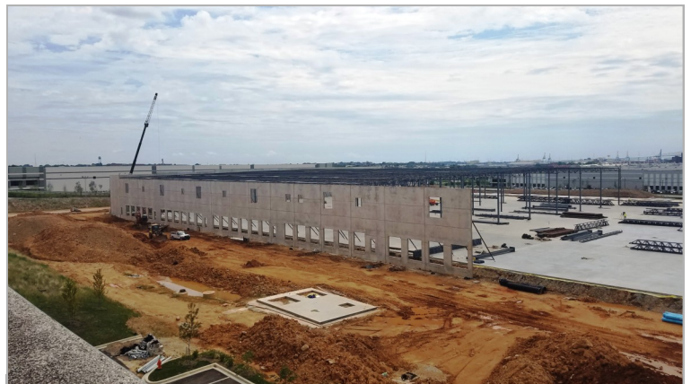
Construction continues at the Port 95 Industrial Park in Southeast Baltimore.
